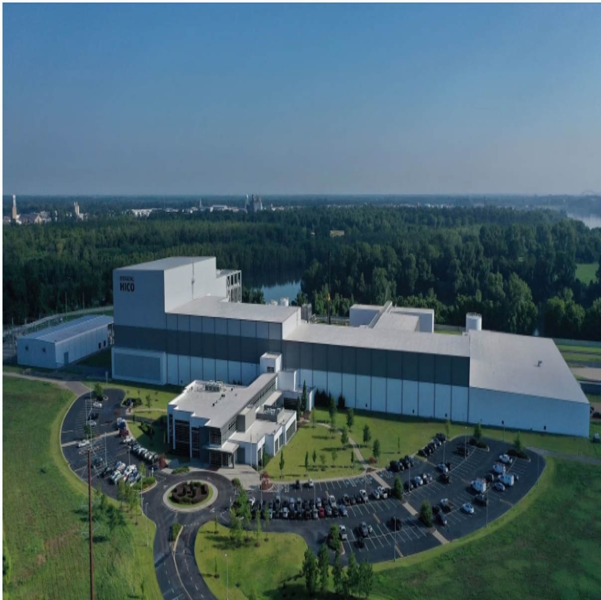
Hyosung Heavy Industries is expanding transformer manufacturing capacity at this Memphis plant not far from where xAI needs a transformer for its giant data center. Photo courtesy of Hyosung
